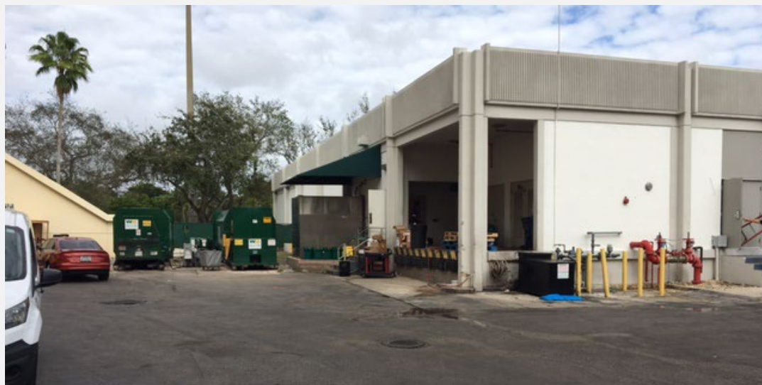
Parking along driveway is not permitted; this is a Fire Lane.
